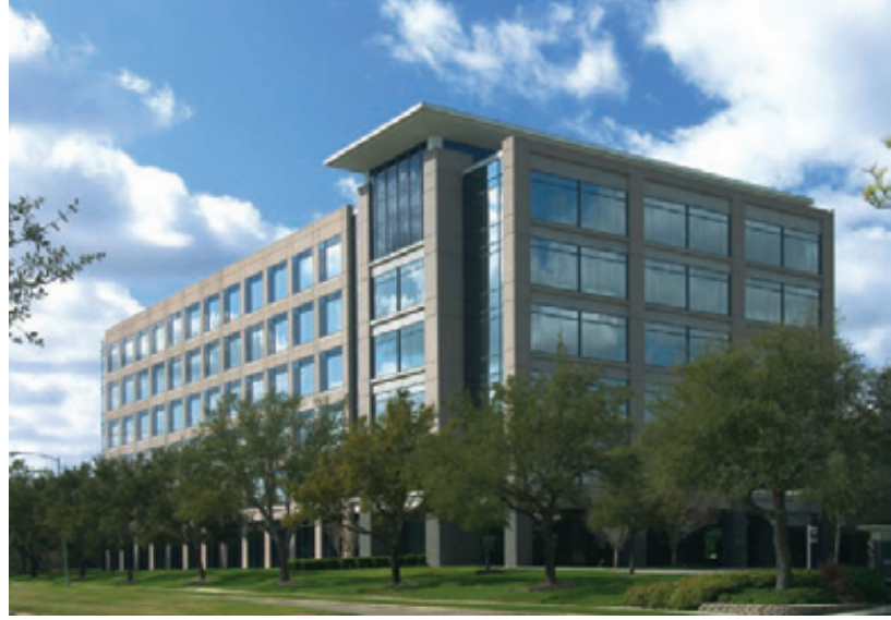
Cabot Oil & Gas Corporation headquarters at 1200 Enclave Parkway in the Energy Corridor, has regional offices in Denver, Charleston, and Calgary.
